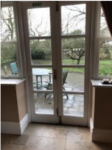
Doors from kitchen to side bbq terrace
